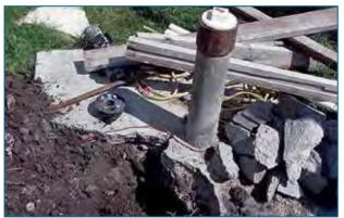
**F**<sub>igure</sub> **59.** The slab around this well is not sufficient to prevent surface contaminants from entering the aquifer. (Source: *Plugging Abandoned Water Wells,* Bruce Lesikar and Justin Mechell, 2010.)
