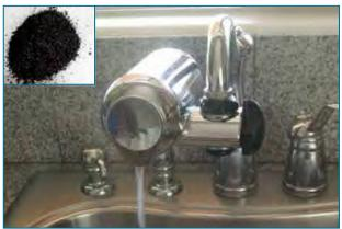
**F**<sub>igure</sub> **54.** An activated carbon point-of-use treatment installed on a faucet; the carbon media is shown in the photo insert.
