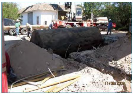
**F**<sub>igure</sub> **49.** Leaking underground gasoline storage tanks are a common source of groundwater contamination.
